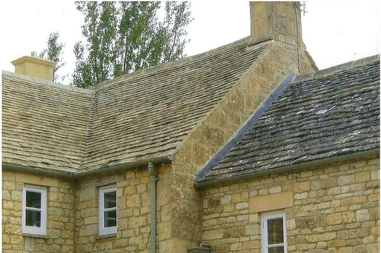
Cardinal roof (left)
